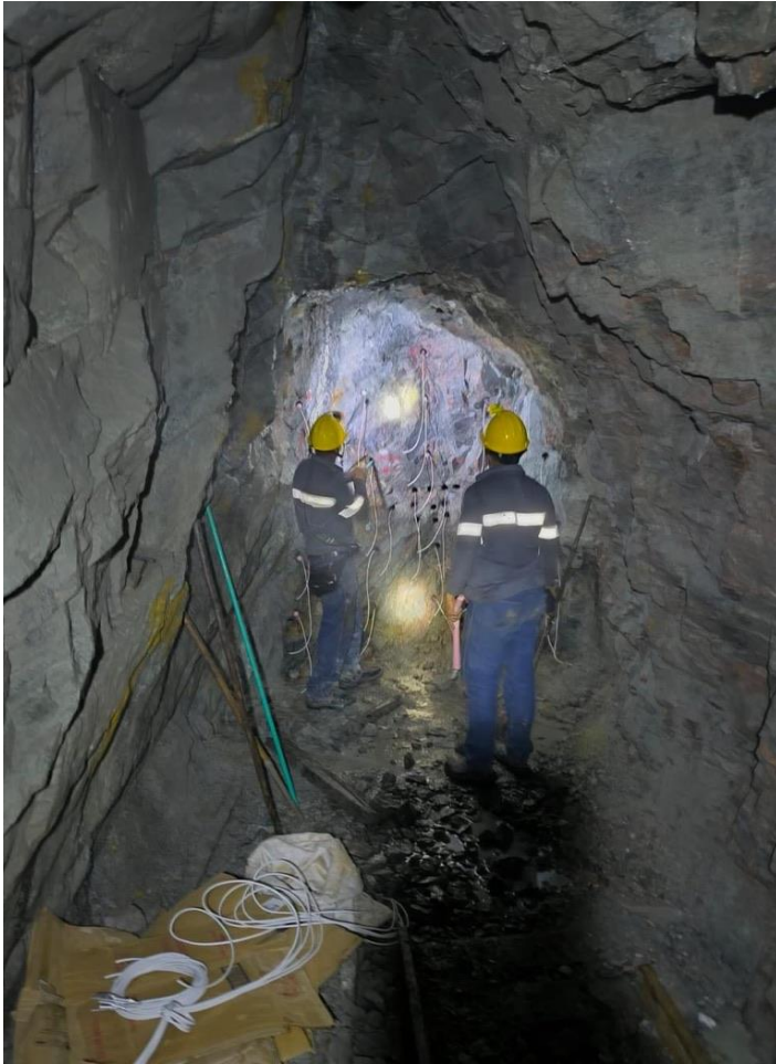
Development Drive Wired for Blasting
